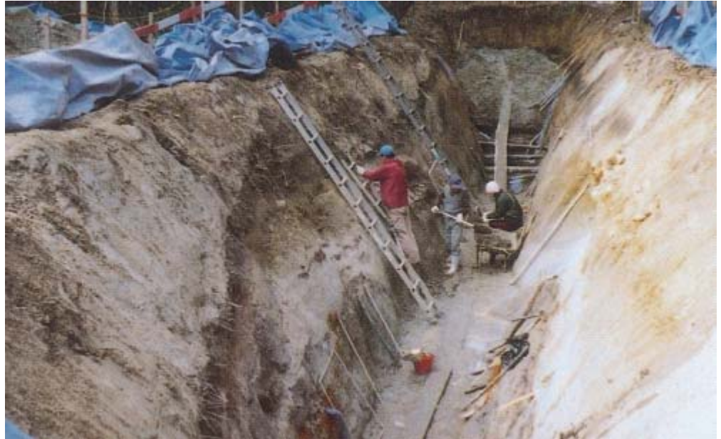
Trench excavation survey (Sanageyama Faults, Aichi)
